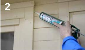
Seal around the outer perimeter of the frame where it meets the logs of the cabin. Always ensure the bead of silicone makes contact with the frame and cabin logs to provide a good seal.
