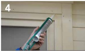
Ensure a bead of silicone is applied around the entire perimeter of the inner frame making contact with both edges of the frame to provide a seal.
