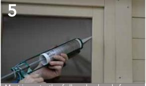
Most importantly of all apply a bead of silicone around the perimeter of the frame where it meets the glass.
