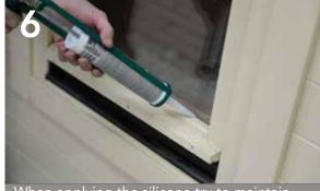
When applying the silicone try to maintain an even pressure on the applicator and use a smooth slow movement as you move the nozzle across the frame.
