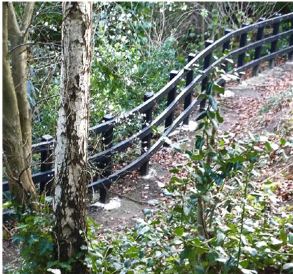
Posts can be anchored to the ground using the same method as timber and steel posts, by concreting, hammered mechanically or surface fixed.
